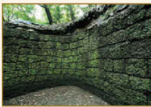
Kiln wall built of tuff blocks The arch-shaped opening and the inner surface of a huge charcoal kiln dome were built tightly with thick blocks of tuff. The structure was sturdy enough to sustain extremely high heat and the weight of a domed ceiling made of clay.
