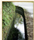
Yoshino Leat Excellent construction technology was required to build a constantly inclined leat over the selected land, because there was little difference in elevation. The 7km leat ending with a steep chute represents a brilliant feat and is testament to the high levels of construction technology at the time.
