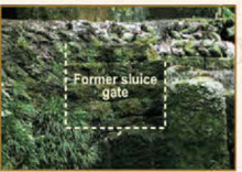
Former sluice gate The sluice gate was moved from time to time. The present one was constructed in the Taisho period (1912-1926). The one used earlier is on the left of the cut in the bedrock of the former dam and covered with stones.
