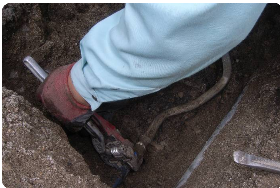
鉛製給水管の取替
