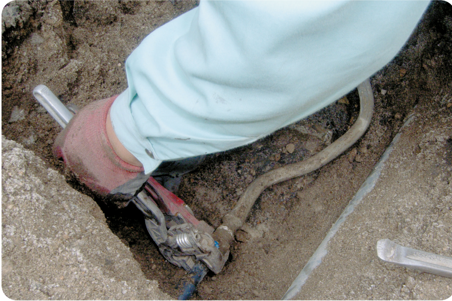
鉛製給水管の取替
